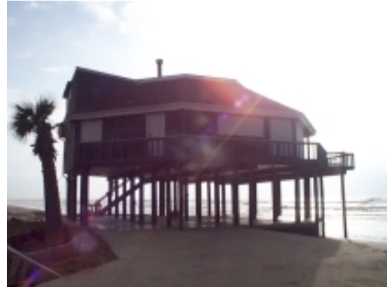
FIGURE 3. As a result of erosion, this oceanfront house is now on the beach.
